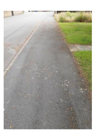
Aesthetic failure due to visible moss, grass or overgrown vegetation and requires cleansing treatment
