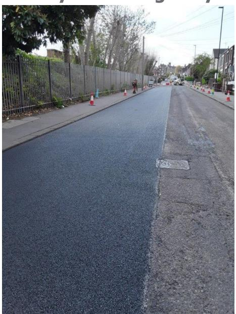
Heely Bank Road – Treatment to one half of carriageway due to failed section data. Other half shows visible defects but does not trigger contract failed section.
