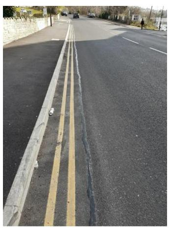
Edge – edge failure – often highlights an unrestrained edge or work undertaken by third party but in acceptable condition
